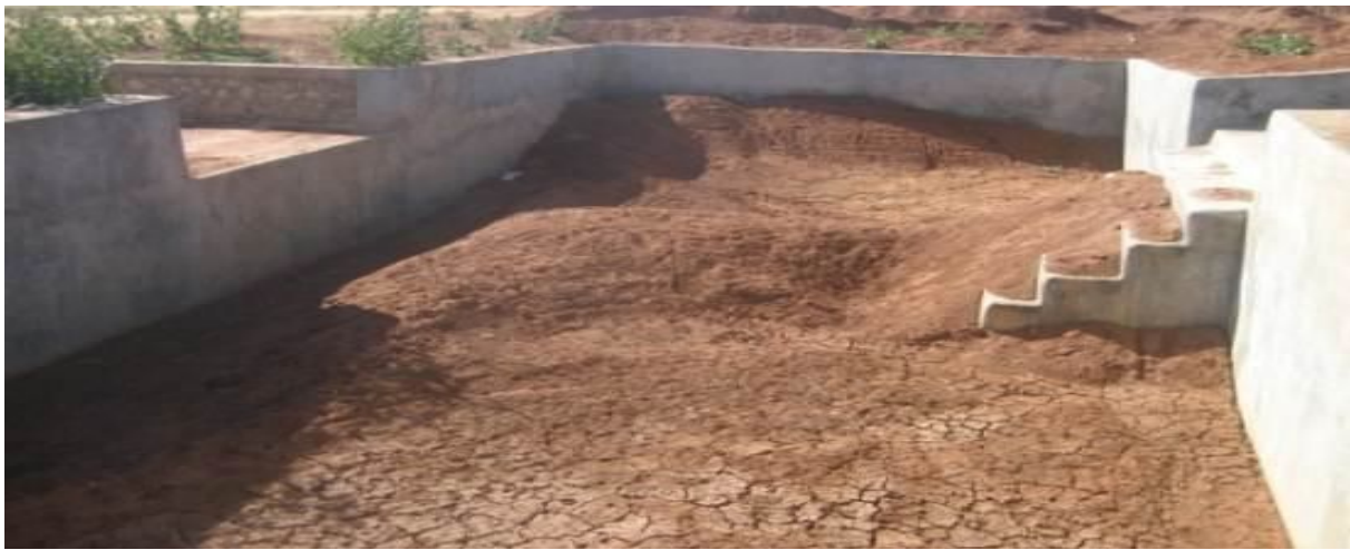
Fig 3.2 - Siltation of Dam in Lupane district
